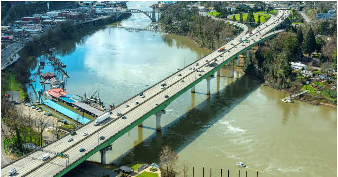
The Abernethy Bridge is one of the nine I-205 bridges to be upgraded or replaced as part of ODOT's I-205 widening program.
